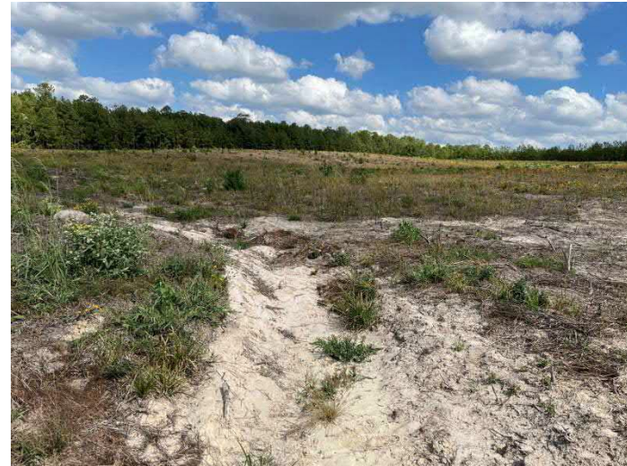
View of Swale 2
