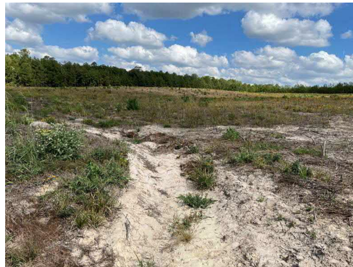
View of Swale 2
